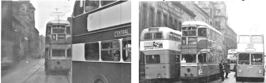
Picture 24. A historic split-second snapshot, taken through ‘my’ side-window in 1174, on the final public service tram journey of all, with us powering half-way down the sharp right-angled junction turn-off curve from London Road into Abercrombie Street, of next-to-last tram 1285 approaching us. It had just reversed there, en-route to Dalmarnock Depot, as our 1174 would itself also do shortly. Never again on any UK city street would two traditional service trams ever pass each other anywhere! 4 September 1962. Photo: author [X1A2]
