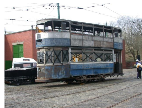
Leeds 345 prior to restoration
